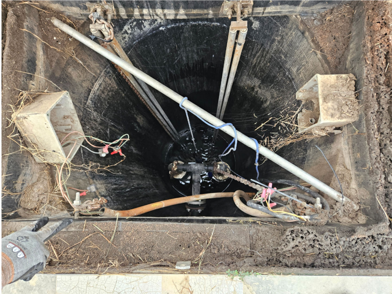
Lime Waste Landfill – Leachate Sump
