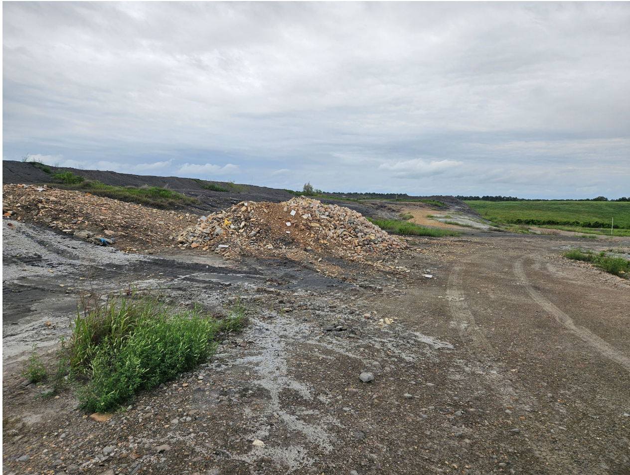
Lime Waste Landfill – Top Deck, Looking South
